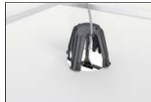
2. Push the spikes into the plasterboard to prevent shifting and disconnect the tool.
