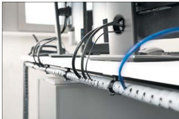
Helawrap - Office Desktop Cable Management.
