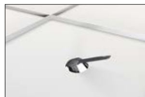
1. Insert the mounting support through the fixing hole.
