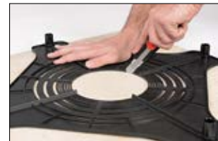
Use the SpotClip-Plate as a stencil to cut the fixing hole into the ceiling plate.
